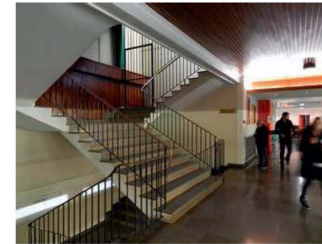
PHOTO ESCALIER PRINCIPAL EXISTANT
