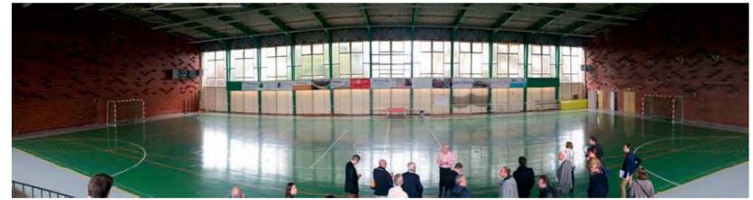
PHOTO GYMNASE EXISTANT
