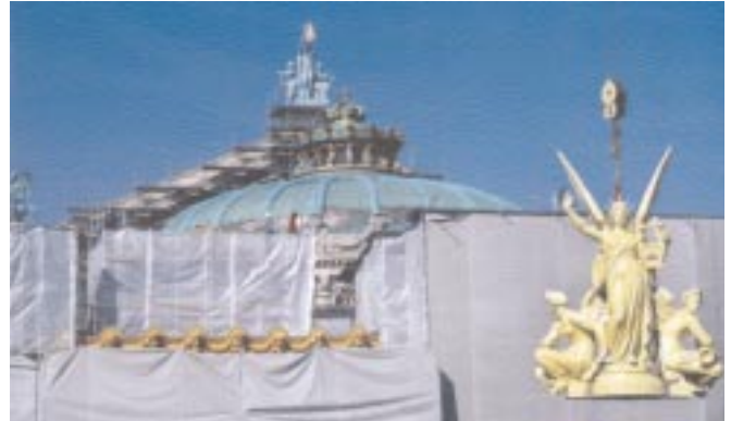
Travaux de restauration du Palais Garnier, 1999-2000, photo © J.-P. Delagarde © J. Moatti
