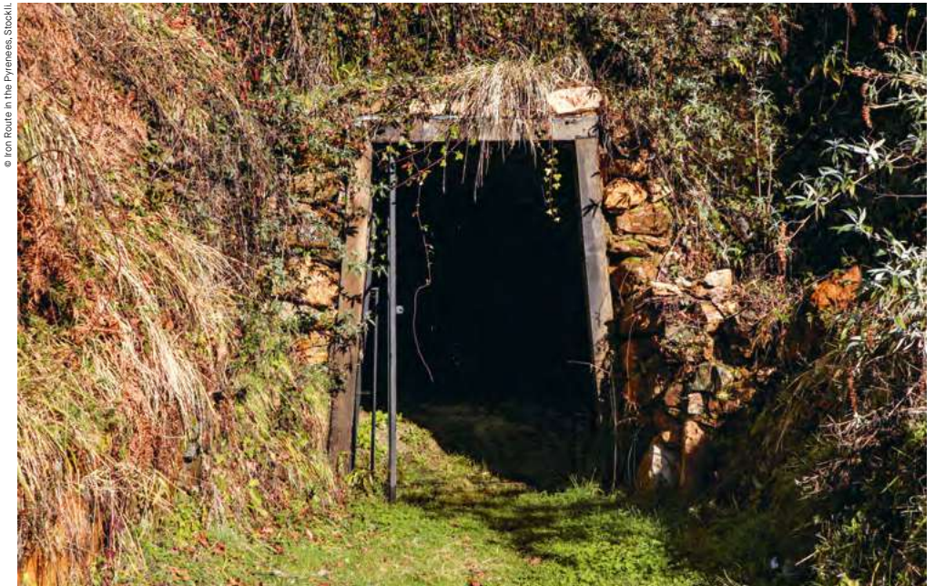
The Baburet mines, an important site in the history of the industrial and social development of the Pays de Nay, Ferrières.
