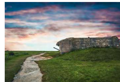
Following the invasion of the USSR and the United States' entry into the war alongside the British, German strategy in the West shifted from offensive to defensive. Hitler ordered the construction of a line of fortifications along the western coast capable of repelling any Allied invasion attempt. Construction of the Atlantic Wall began in early 1942.
