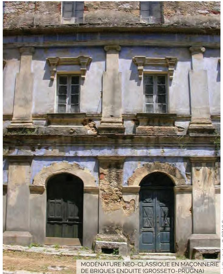
MODÉNATURE NÉO-CLASSIQUE EN MAÇONNERIE DE BRIQUES ENDUITE (GROSSETO-PRUGNA)
