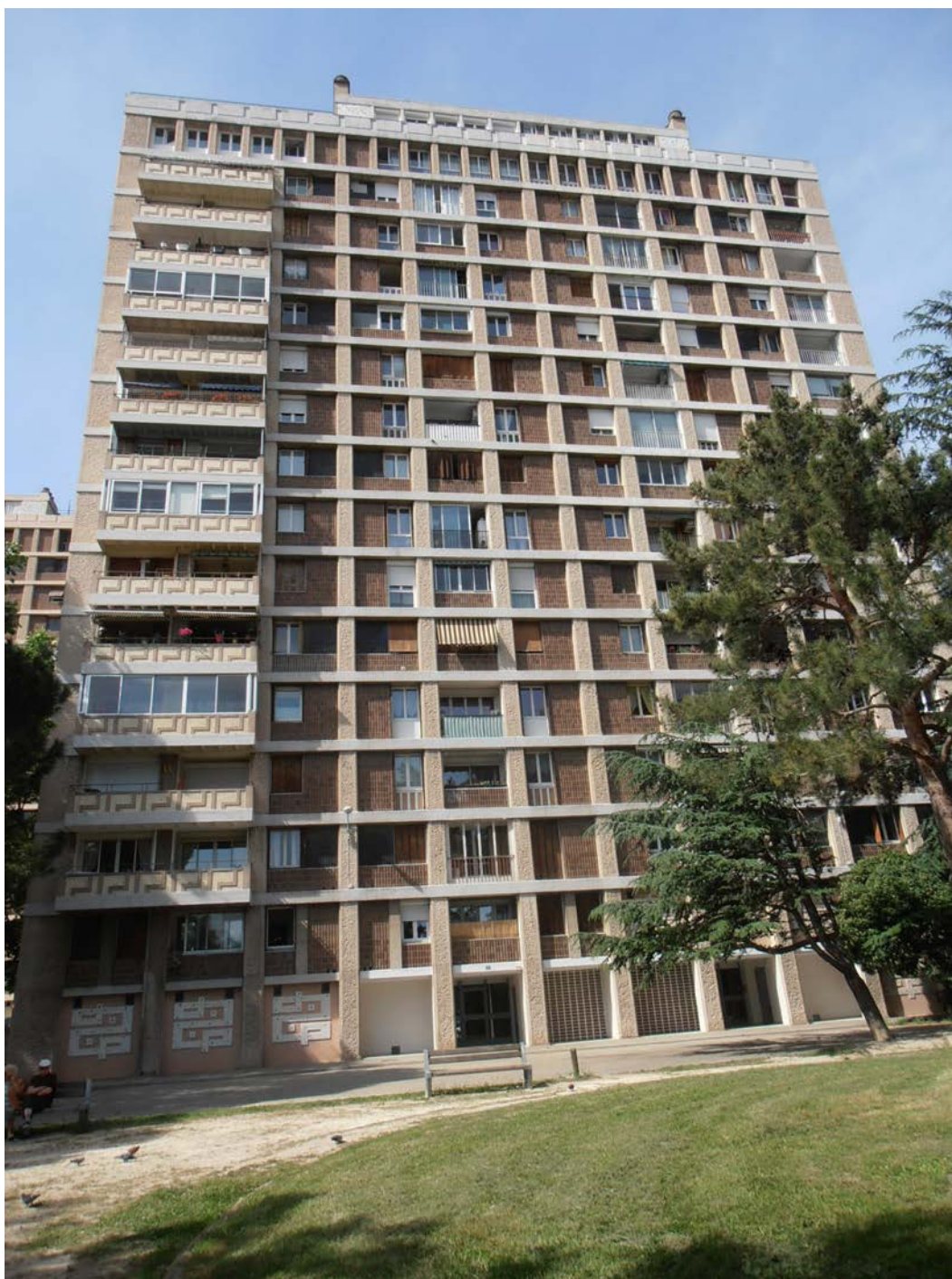
Immeuble Sixte-Isnard, Avignon (84) © DRAC PACA/Architecture
