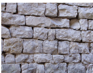
Mur : limousinage (Naves)
