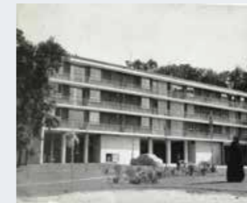
Ardenay District, Palaiseau, 1960 Architect: R. Audigier © D.R.
