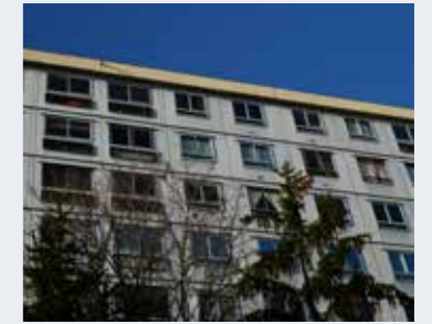
The Prouvé panels, south facade. Date of photo: March 19, 2018 Photographer: Mathilde Padilla © Research Project RFL – Rehabilitation of Light-Weight Facades in 20th Century Housing
