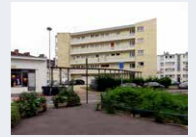
Saint-Lô, Torteron Street Architect in Chief: Marcel Mersier ©Patrice Gourbin
