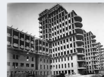
Beaujon Hospital during construction. APHP Archives (1934)
