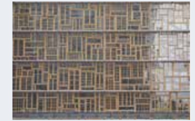
Facade of the European Council in Brussels, Belgium, with recycled chassis-frame base, 2016 Architect: Philippe Samyn © Pierre Belli-Riz
