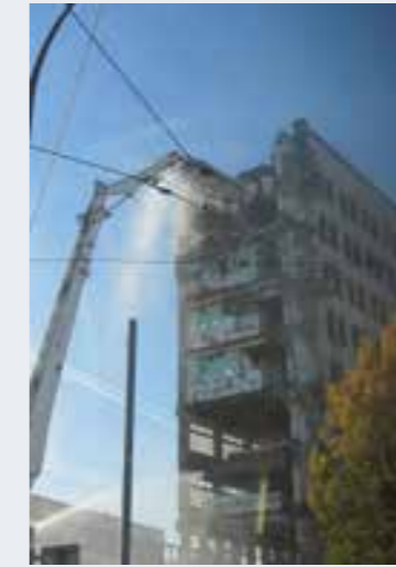
Demolition of a building in Grenoble, 2006 © Pierre Belli-Riz
