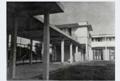
Port-Louis School Group Architect: Ali Tur Architecture d'Aujourd'hui , March 1936, p. 103. © D.R.
