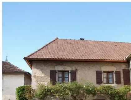
Tuile plate pressée (65 unités/m²).
