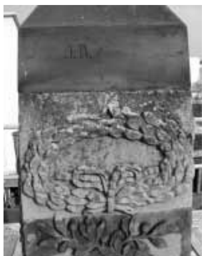
Figure 5 : Too coarse grained
