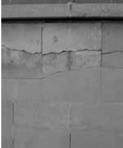
Figure 1 : Shrinkage
