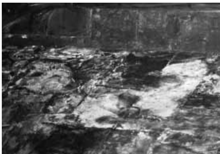
Figure 8 : Springtime condensation on cold walls at Castel del Monte (Southern Italy). When the warm and humid Sirocco wind blows at the end of the cold season, walls cover with water droplets, here evidenced by the use of flash light. For surfaces perpendicular to the flash light, the light crosses the droplets, which then appear invisible (on the right). For nearly parallel surfaces, light undergoes multiple reflections inside droplets, which then appear brilliant white (on the left).
