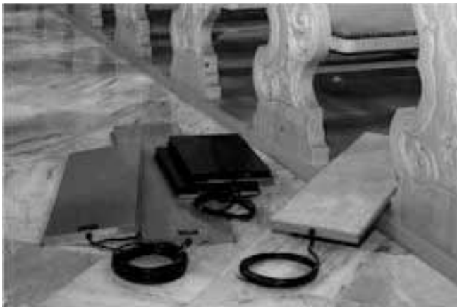
Figure 6 : Electric pew heating. Thermo-electric heating foils can be inserted into pews themselves to avoid visual impact (by courtesy of HTS EGGER & GRUTSCH KG, Austria http://www.thermotex.at ).
