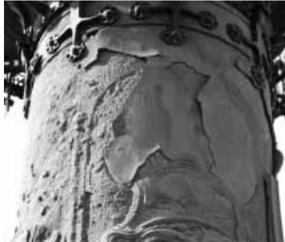
Figure 2 : Lack of adhesion
