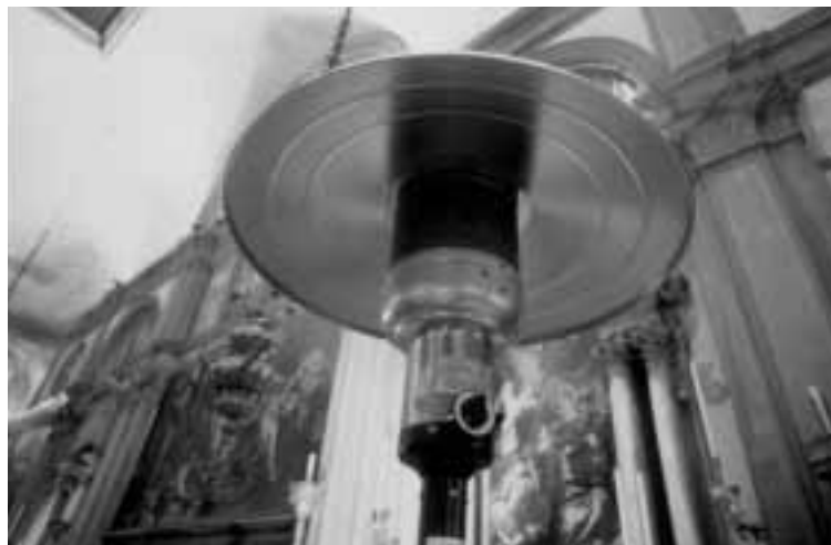
Figure 4 : Direct gas burning (catalytic or mantle stoves) releases dangerous moisture that may condense on cold walls.
