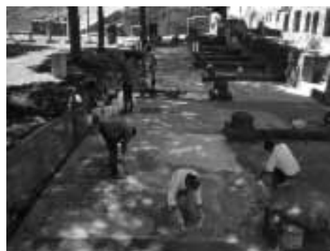
Figure 8 : Ostia Antica Maintenance of monuments by using traditional materials and techniques.
