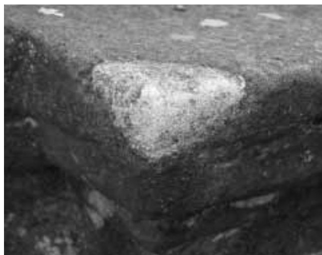
Figure 6 : Salt efflorescence
