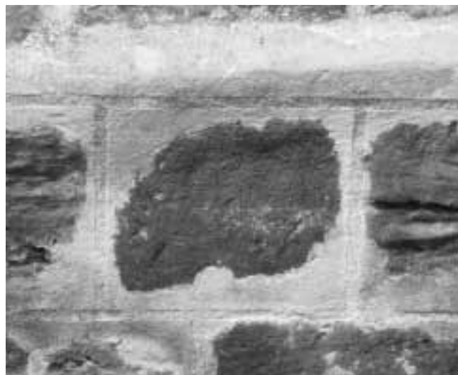
Figure 4 : Biological aggression (more biological layers than on original stone or less biological layers than sandstone).
