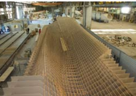
Photo Drassm, S. Cavillon
